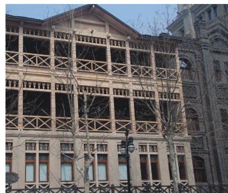
This hotel has recently had its entire facade installed – manufactured of course with mitred corners and jointed with the Hoffmann Dovetail System.
